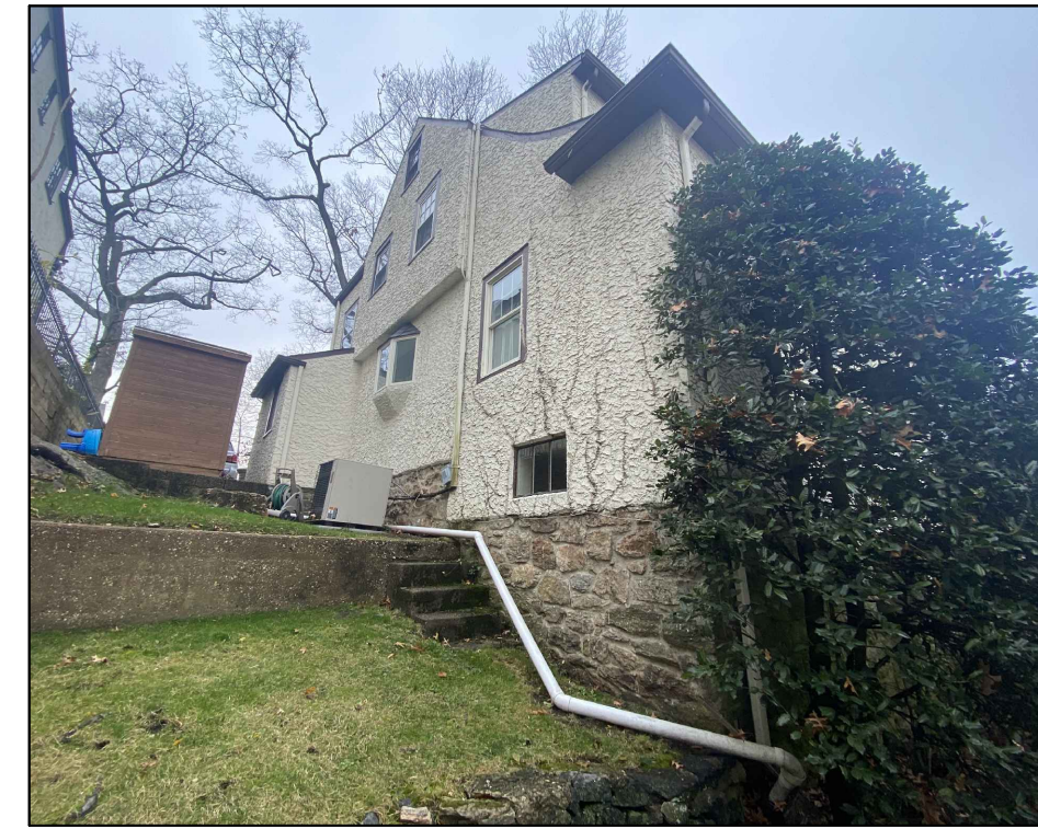
3 - 10 HALL AVE REAR
