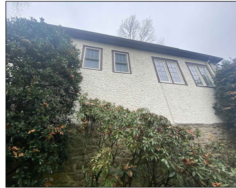
2 - 10 HALL AVE LEFT
