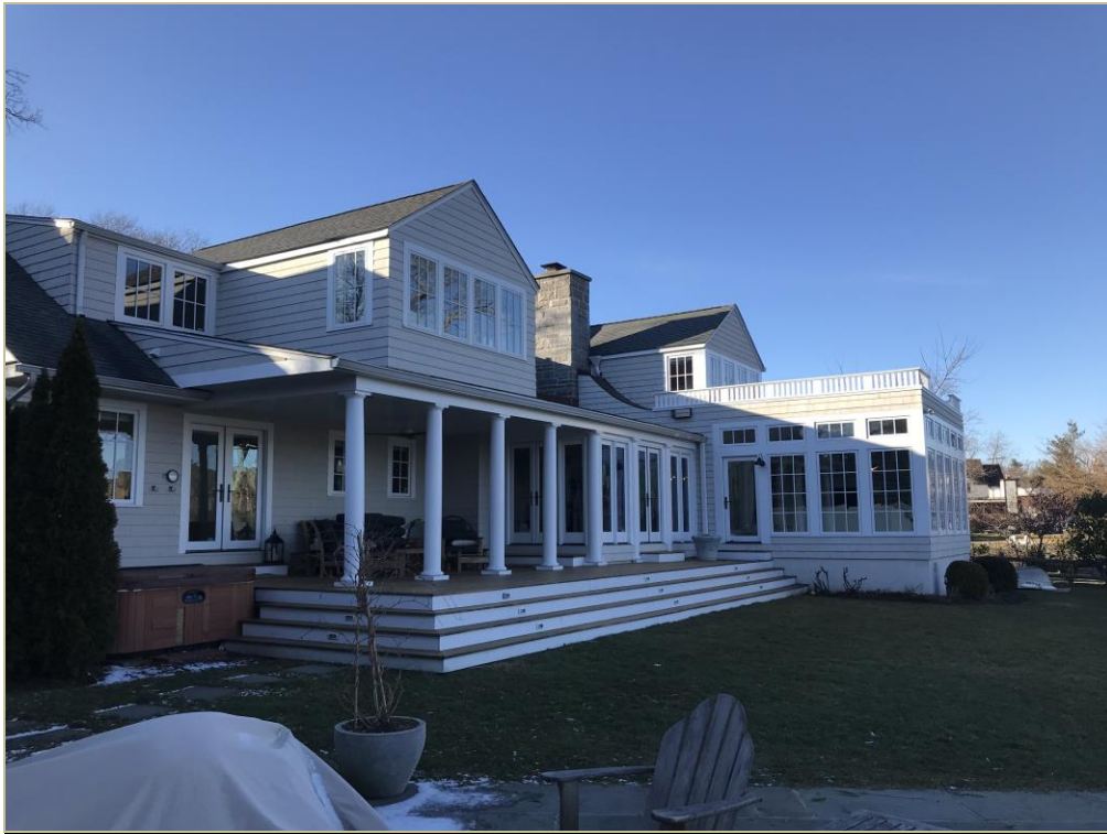
Figure 3 – Rear façade of 15 Bishop Place
