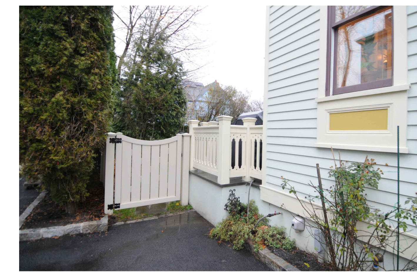
D Existing Pool Fence/Evergreen Hedge at Driveway Looking NE from Driveway off Helena Ave NOTE: Gate to be replaced/relocated to meet pool barrier code requirements. Proposed fence style to match existing.
