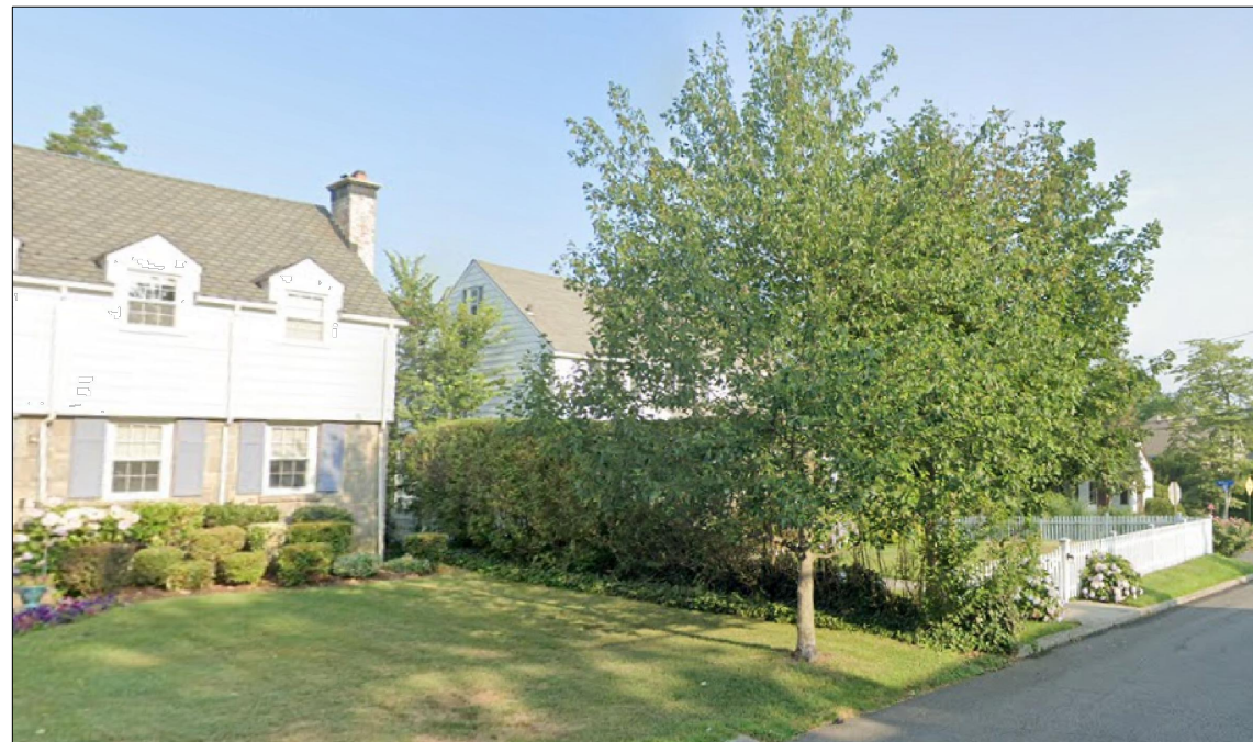
LOOKING NORTH ON KANE AVENUE, PANEL ARE ON REAR ROOF AND NOT VISIBLE FROM STREET
