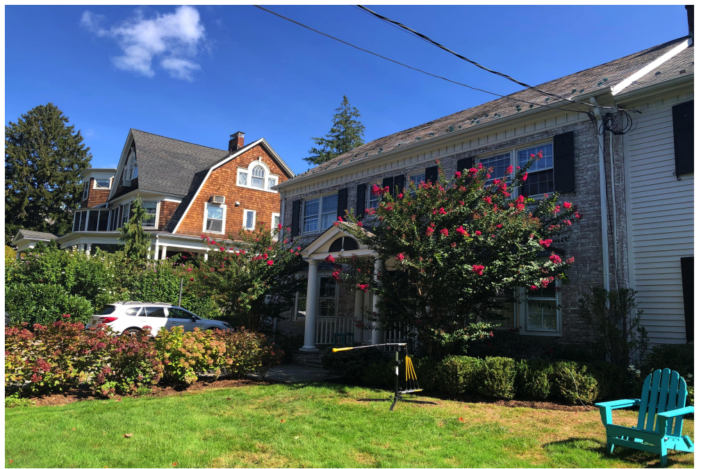
FRONT ELEVATION FACING NORTH
